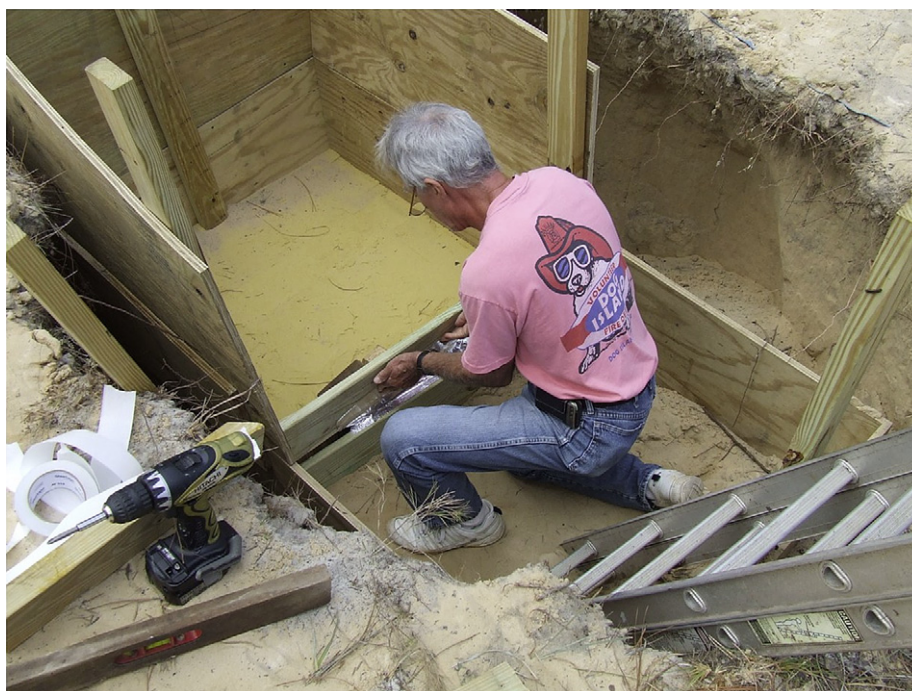
Fig. 2. Construction of the layered sand column within the plywood box. Beginning at 2 m depth, different colors of sand were layered and packed. The open side of the box was closed with boards as the level of sand rose. The yellow sand layer is shown in place here. Once complete, all sides around the box, and the work pit were refilled with sand. (For interpretation of the references to color in this figure legend, the reader is referred to the web version of this article.)
